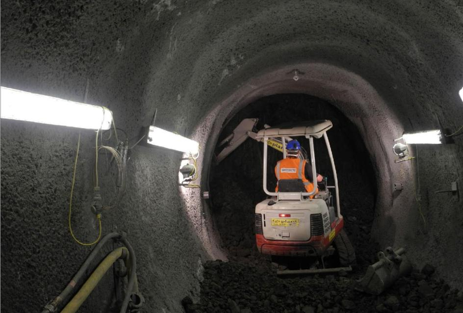
Works were to construct a new cable tunnel and shaft and tie into the existing Liverpool St underground station.
